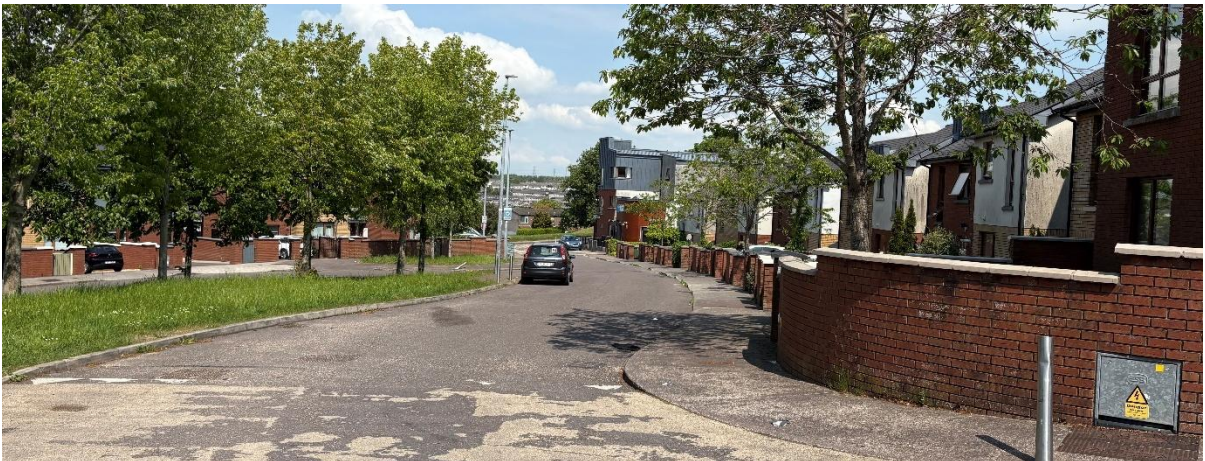
Plate 1.5.6 Adjoining Gleantrasna housing estate to the north of the subject site
