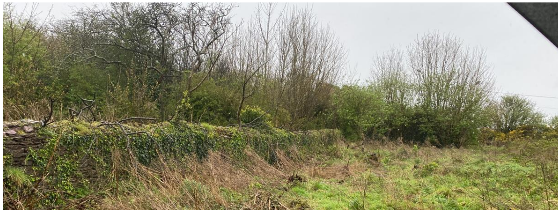
A: North boundary: Vegetation and stone wall
