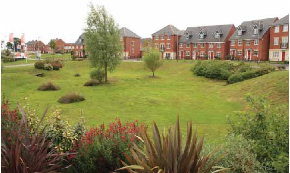
Figure 3.11 Detention Basin Example (ref: SUDS Manual)
