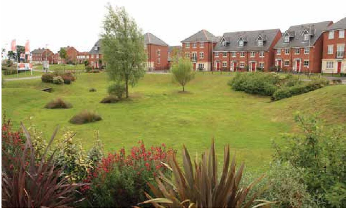
Figure 3.12 Detention Basin Example (ref: SUDS Manual)
