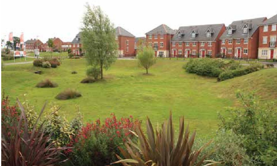
Figure 3-9 Detention Basin Example (ref: SUDS Manual)
