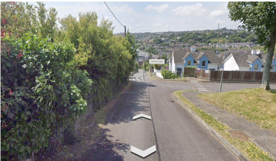
Figure 3-24: Popes Road/Popes Hill Intersection © Google Earth Streetview - View from Popes Road (Westbound)
